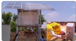
SPV Water Pumping System for drinking water
